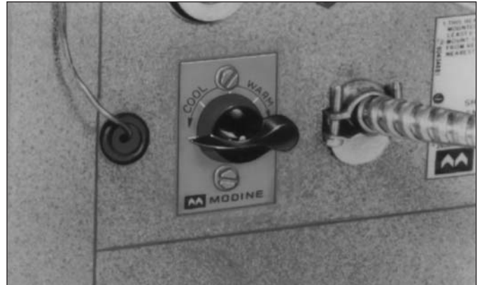
Figure 7.1 Unit-Mounted Thermostat
